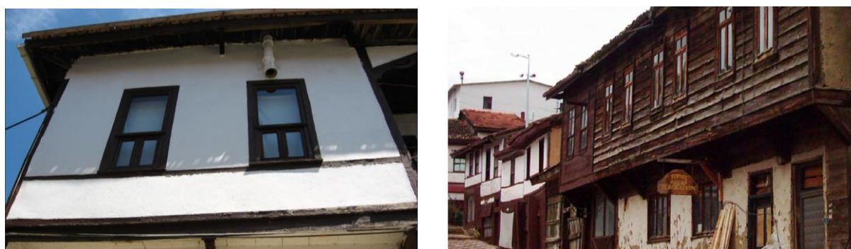
Figure 14. Example of overhangs.
