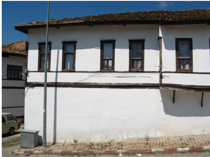
Figure 5. An Example of mud plastered application the facade of the building.
