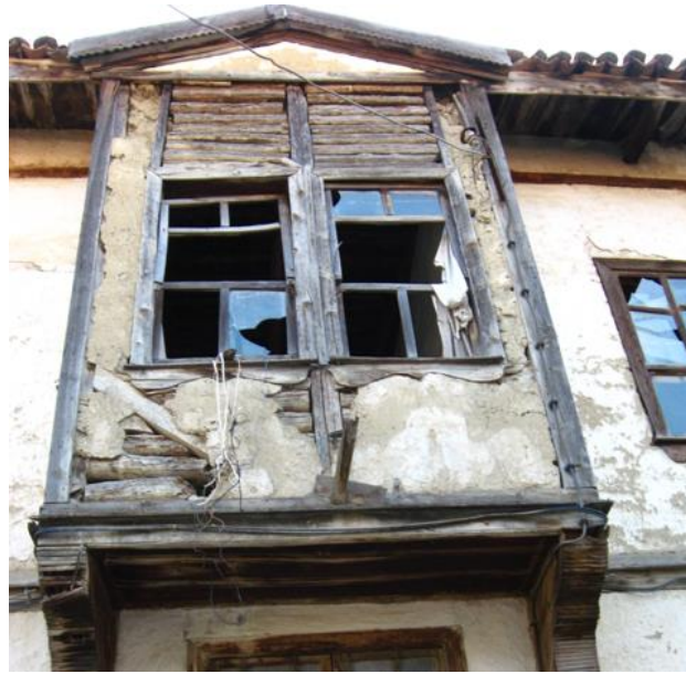
Figure 6. An Example of the bagdadi plaster technique.
