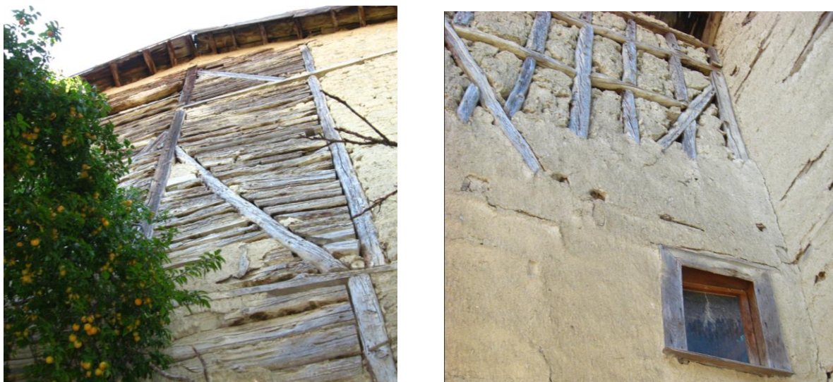
Figure 3. Example of wall detail of wooden structure.
