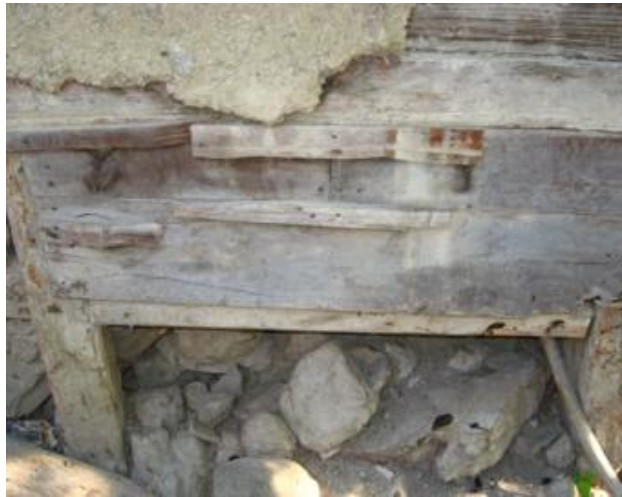
Figure 2. Example of rubble stone foundation.
