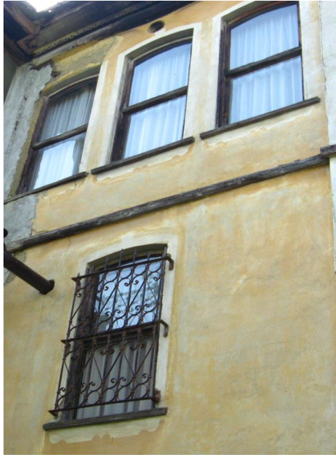
Figure 19. Example of arched windows.
